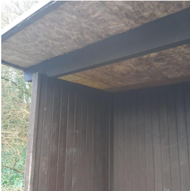
Internal roof OK
