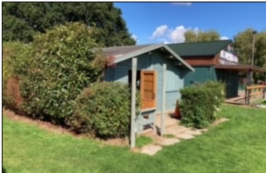
A reminder of the current state of the Cuckoo Shed. The roof is leaking in places. Light and power are not connected. We have not been able to inspect the condition of the windows.
